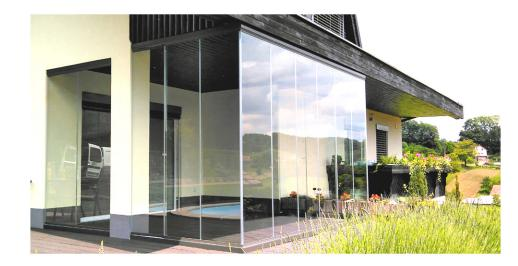
Panels can move through corners with angles between 90° and 270°.
